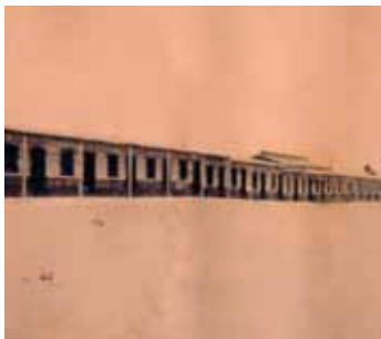
Street of the Worker's Camp, c.1930.
