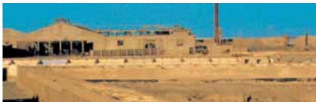
Single worker's quarters on the West and South end of Chacabuco.
